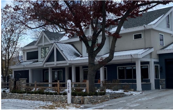
Front elevation. Photo by FWesterkamp Design Inc.
